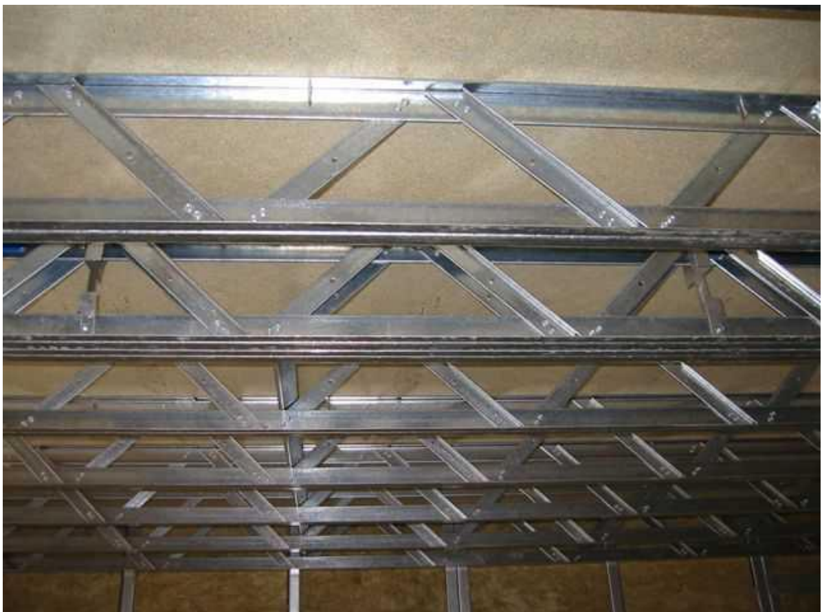
FIGURE 25 - LATTICE WEBBED "I" JOISTS
