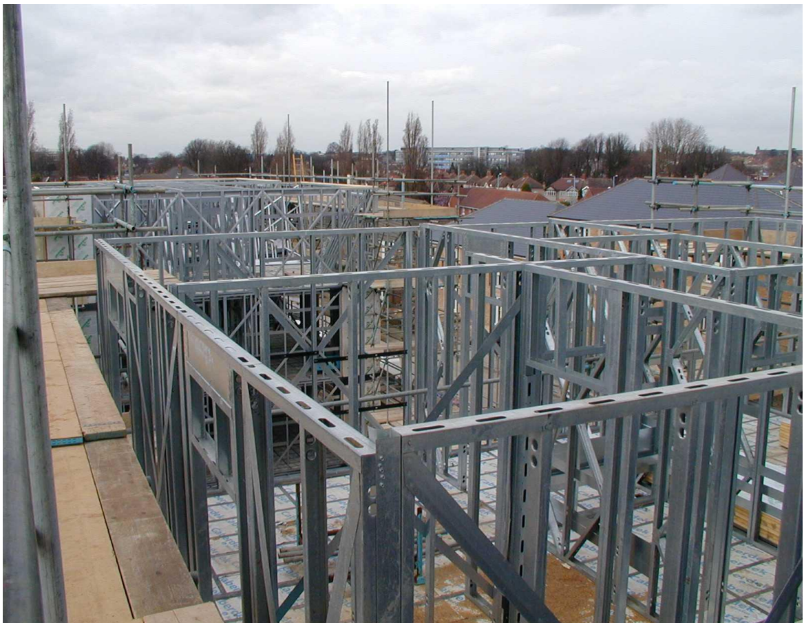
FIGURE 23 - STEEL FRAMES ASSEMBLED TOGETHER
